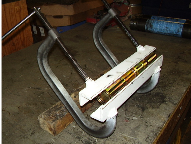
Figure 3: Aligning the Components to be Welded
