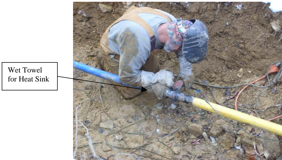
Figure 4: Proper Setup with Heat Sink
