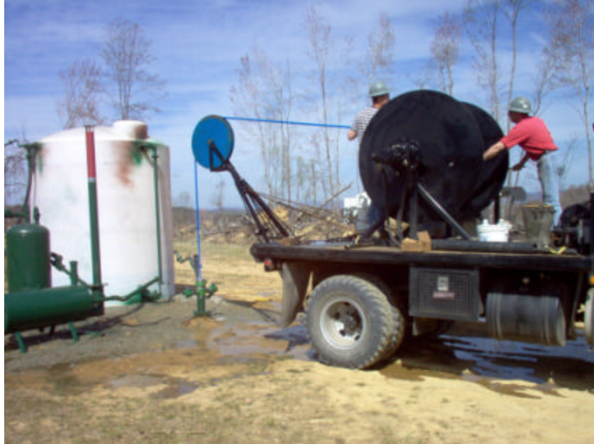
Thermoflex ® tubing installation utilizing a direct drive spooling unit.
