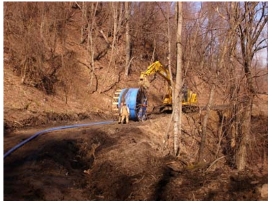
Moving Spool Along Right of Way
