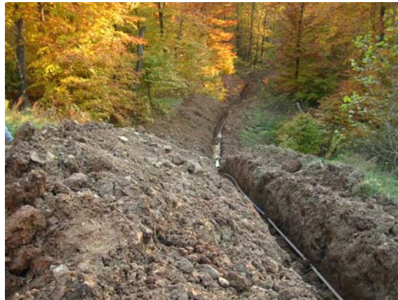
Typical Backfill Material
