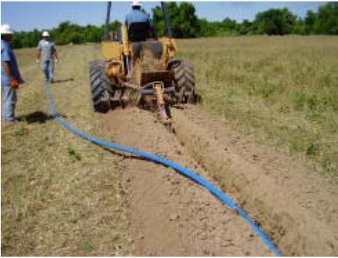
Ditch Witch Trenching
