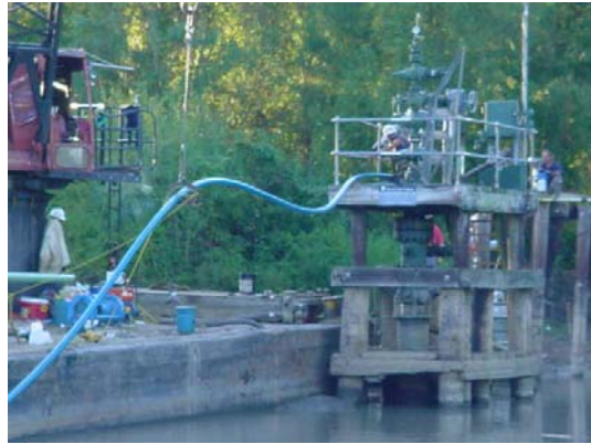
Pulling Through Line from Offshore Well
