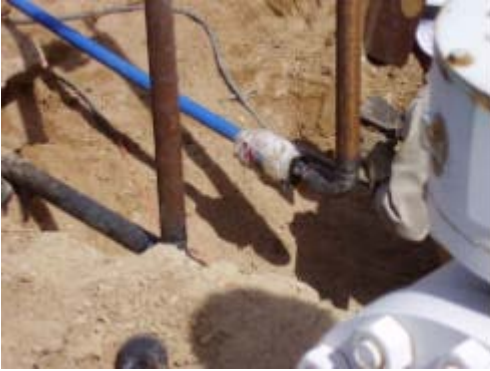
Using a Wet Rag for a Heat Sink
