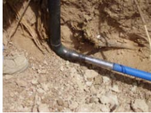
Final Assembly to a Riser
