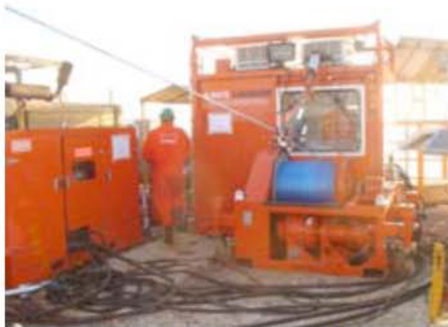
Figure 1: Pulling Rope and Winch
