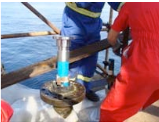
Figure 6: Flange Termination
