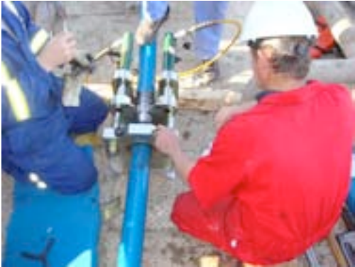
Figure 4: Splicing Tubing Together
