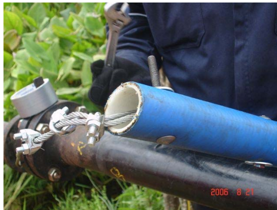
Pulling without a coupling or pulling cone
