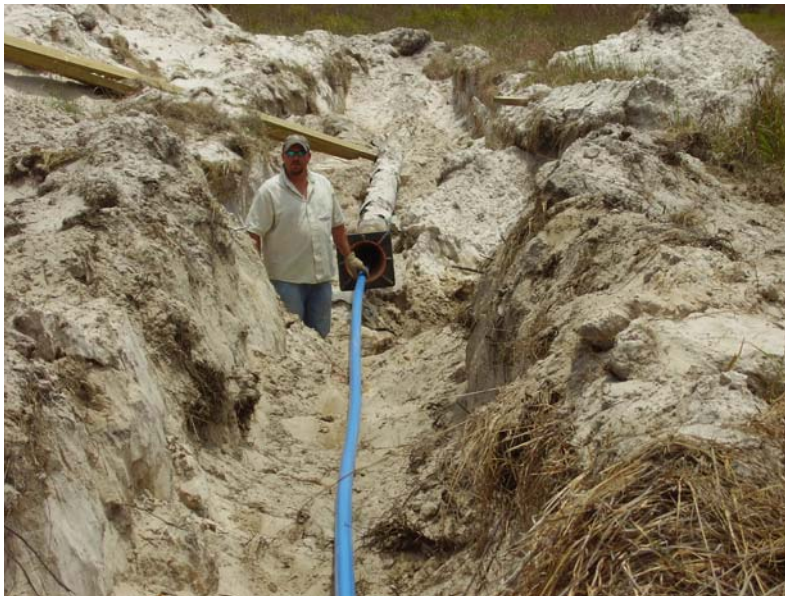
Onshore to offshore straight length before entering existing pipe
