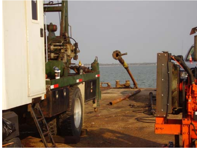
Removing the Riser and lifting the Existing Pipeline onto a Barge
