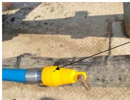
Pulling Cone Attached to a Thermoflex Termination Coupling
