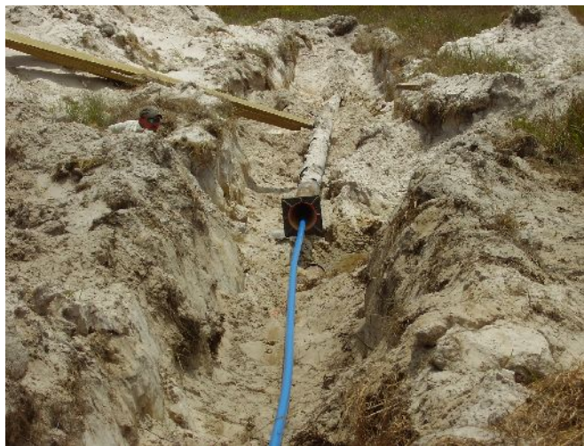
Figure 3: Pulling through the line
