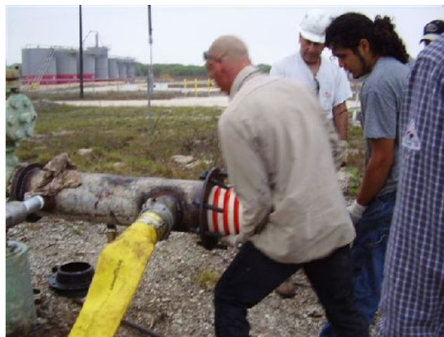
Setting the Pig in Place
