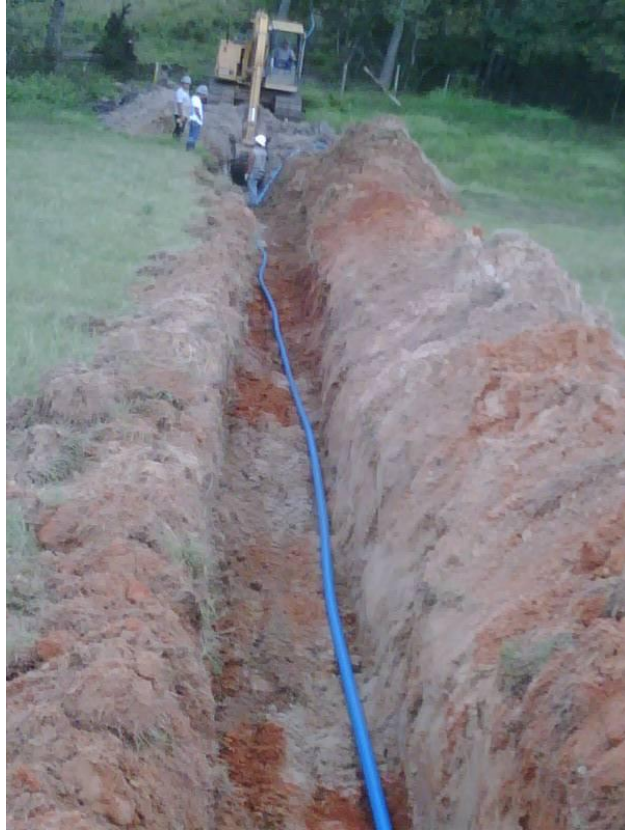
Figure 1: Layout of the Pipe in the Trench
