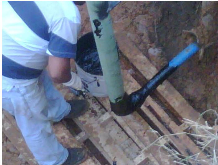
Figure 3: Coating the Weld
