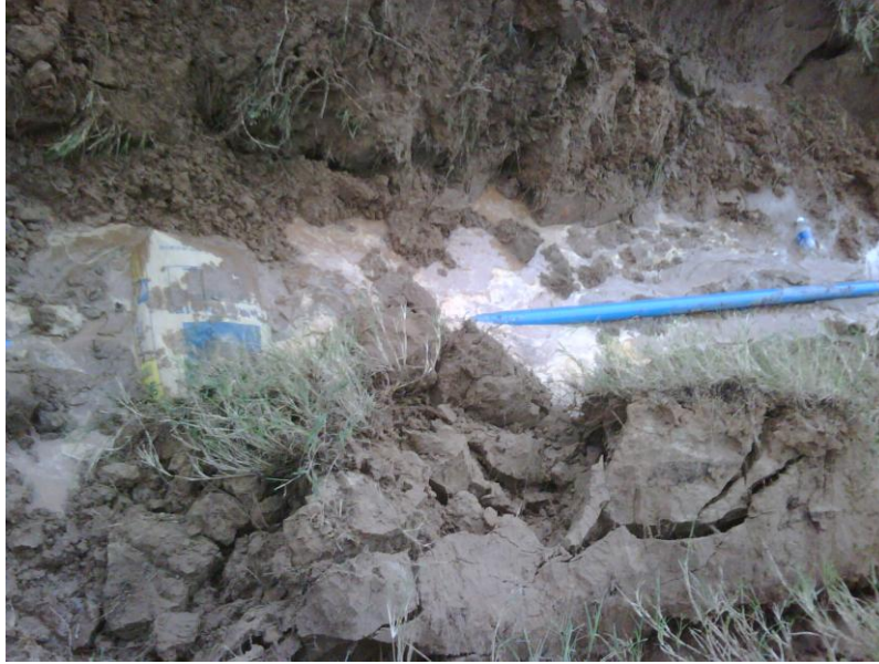
Figure 2: Concrete bags on top of the pipe
